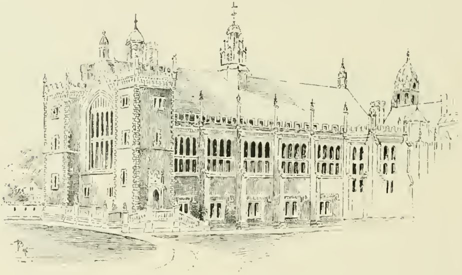
EXTERIOR OF NEW HALL, LINCOLN'S INN.
